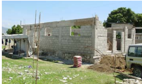
Construction is underway for a Worship Center
